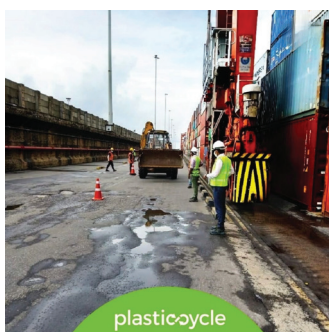
PMAC road resurfacing project at SAGT
